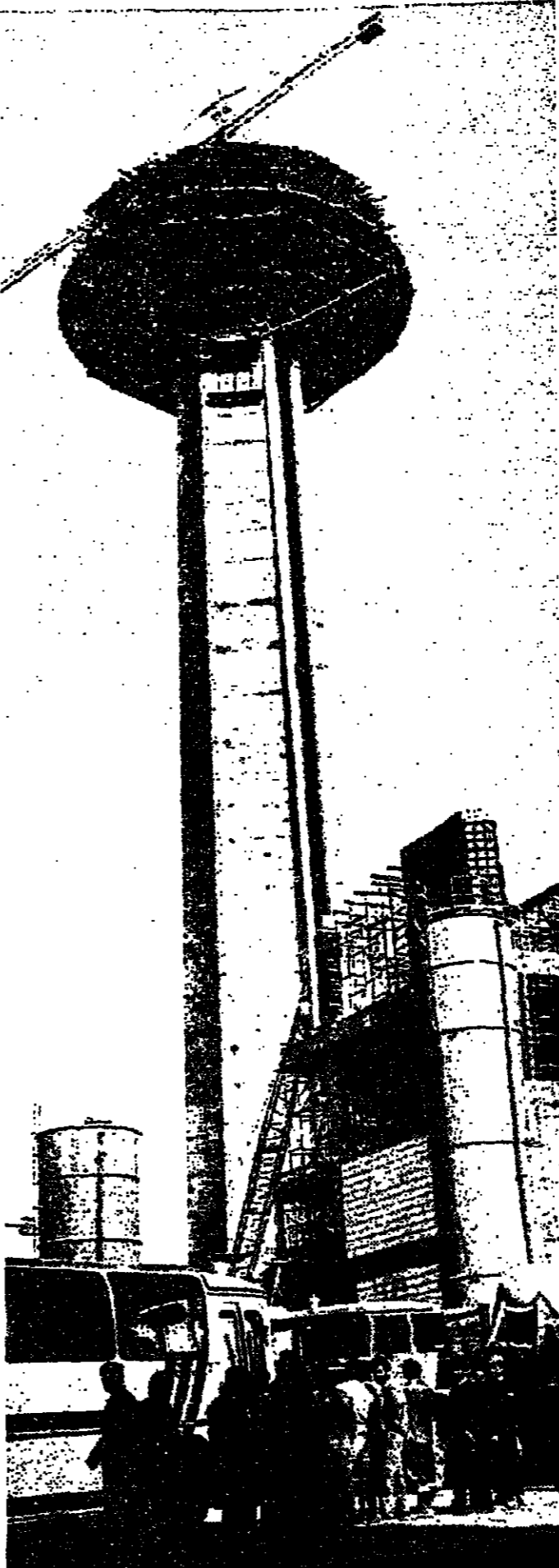
The Cankaya Tower, Ankara, now under construction
